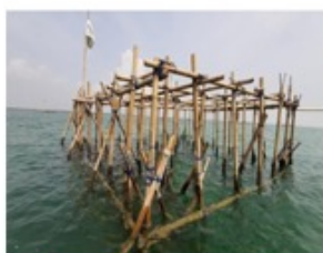
Step 1: Construction Bamboo and rope construction for green mussel culture seawards mangroves greenbelt
