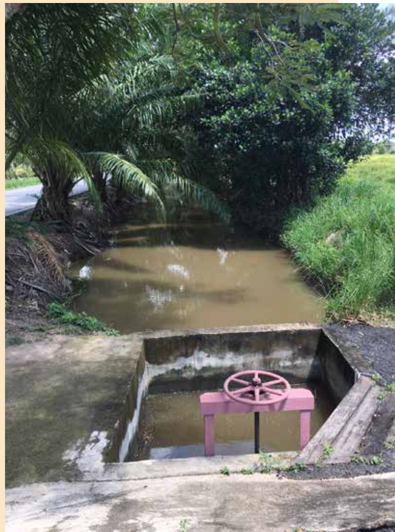
The furrows behind the lock system which connected them to the main river canals.
